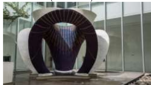
Fig. 14 The total weight - 55 kg (121 lbs) size -50 m2 (538 ft2) in. lightweight shuttering.
