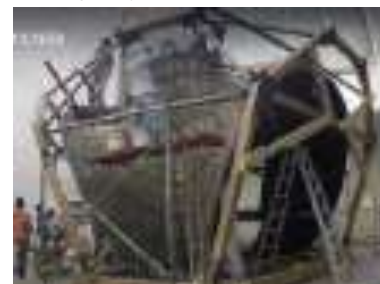
Fig. 13 knitted fabric, a technology KnitCrete, which was covered with 5 tonnes (5.5 US tons) of concrete.
