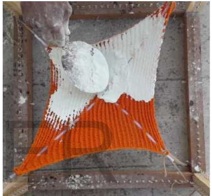
Fig. 73 Top View Applying cement paster
