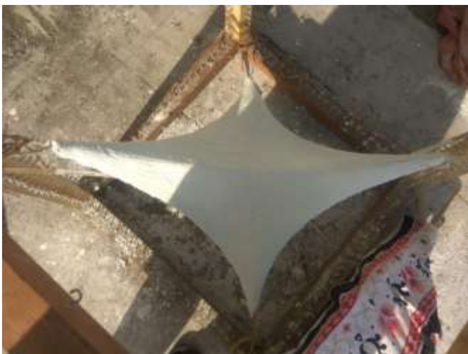
Fig. 74 Top View After applying cement sand mortar
