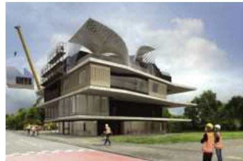
Fig.11 Visualization of the preliminary design for NEST, with HiLo constructed at the top corner. EMPA and Gramazio & Kohler.
